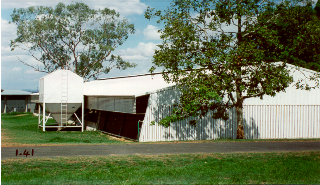
Plate 1 The experimental ridge ventilated gable shed looking from the NW corner
